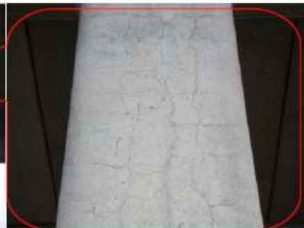
Fig. 5.12 2#reticulated cracks in the pier body of the pier (2)
